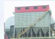
KLMC低压脉冲长布袋袋式除尘器
